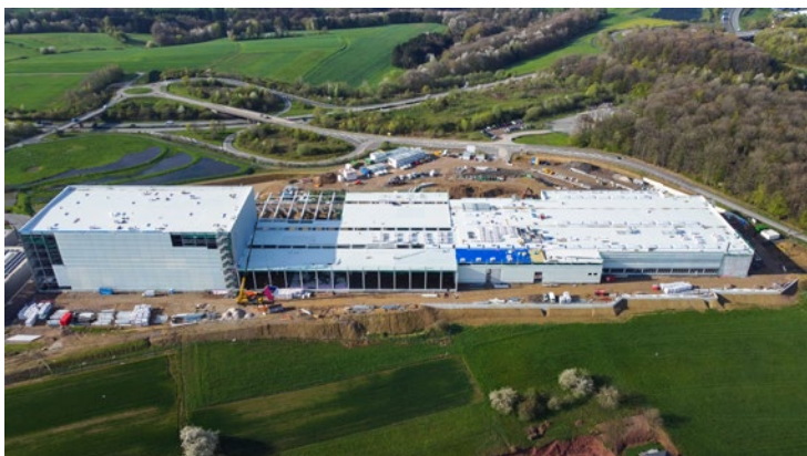
Construction site Progroup Board PW15, date: April 2023 Petersberg, Rhineland-Palatinate, Germany
