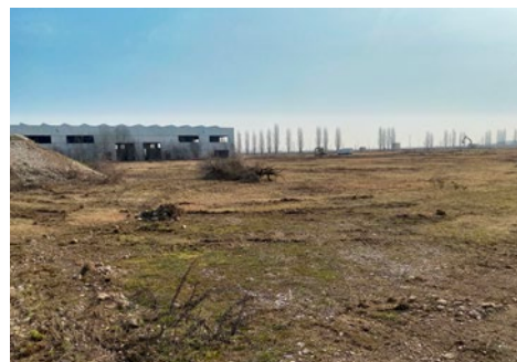
Construction site Progroup Board PW16, date: March 2023 Cessalto, Italy
