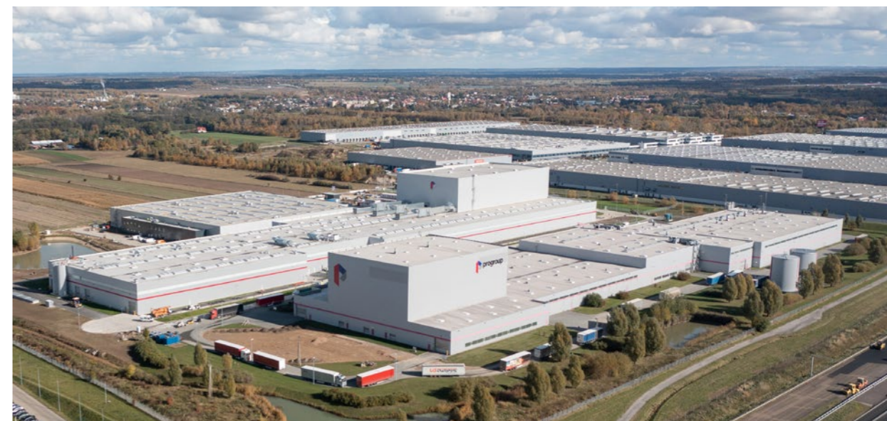
Production site Progroup Board PW07 and PW14, date: March 2023 Stryków, Poland
