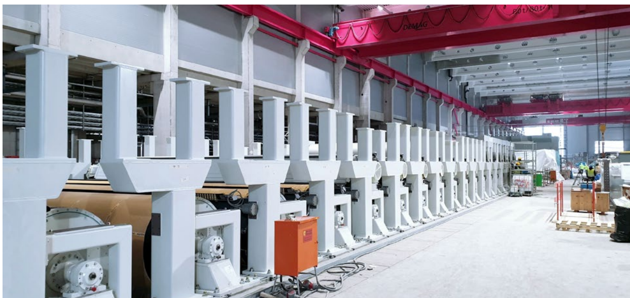
Construction site Progroup Paper PM3, date: 20.01.2020 Sandersdorf-Brehna, Germany
