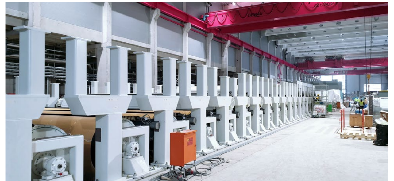
Construction site Progroup Paper PM3, date: 20.01.2020 Sandersdorf-Brehna, Germany
