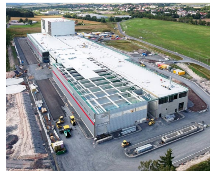
Progroup Board PW13 plant Eisfeld, Germany
