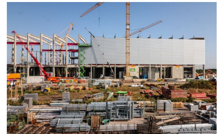
Construction site Progroup Paper PM3, date: 01.08.2019 Sandersdorf-Brehna, Germany
