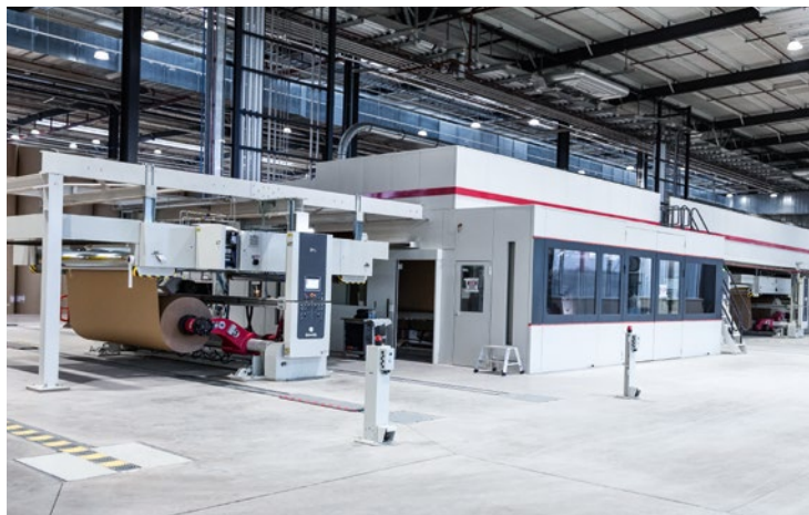
Start of our new corrugated sheetboard production site Ellesmere Port, United Kingdom
