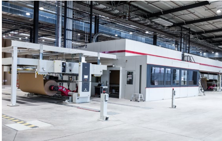
Start of our new corrugated sheetboard production site Ellesmere Port, United Kingdom
