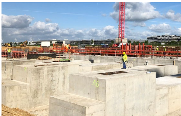
Construction site Progroup Paper PM3 Sandersdorf-Brehna, Germany
