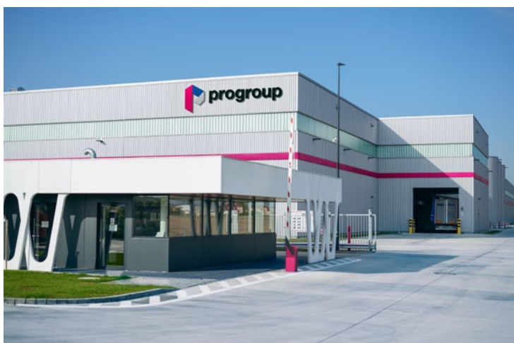
Progroup Board PW10 plant Trzcinica, Poland
