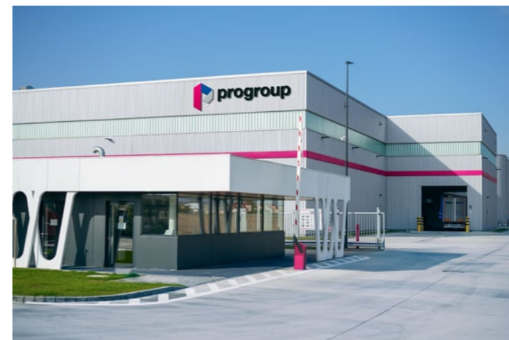
Progroup Board PW10 plant Trzcinica, Poland
