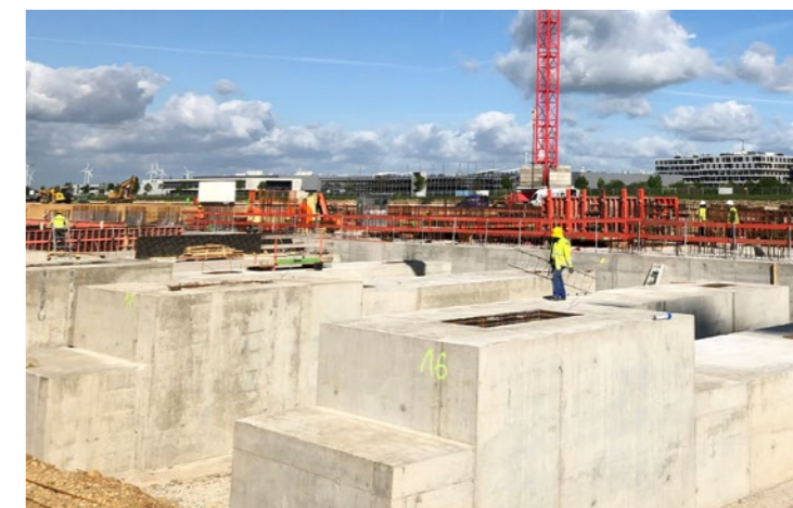
Construction site Progroup Paper PM3 Sandersdorf-Brehna, Germany
