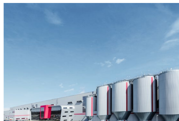
Progroup Paper PM2 plant Eisenhüttenstadt, Germany
