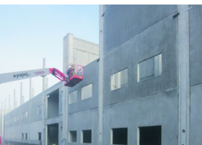
Under construction: PW10 in Trzcinica, Poland
