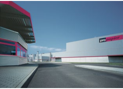
Propapier PM1 plant Burg, Germany
