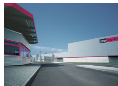
Propapier PM1 plant Burg, Germany
