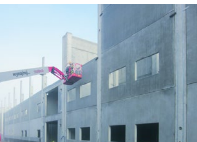
Under construction: PW10 in Trzcinica, Poland
