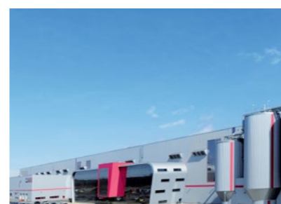
Propapier PM2 plant Eisenhüttenstadt, Germany
