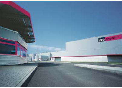
Propapier PM1 plant Burg, Germany
