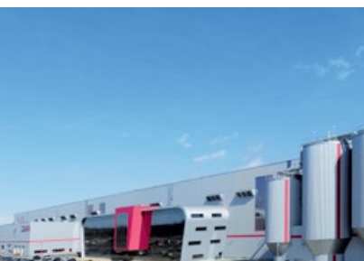
Propapier PM2 plant Eisenhüttenstadt, Germany
