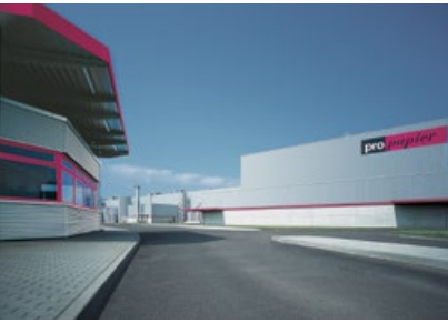
Propapier PM1 plant Burg, Germany
