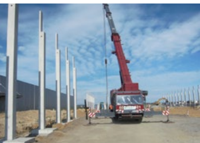
Under construction: PW10 in Trzcínica, Poland
