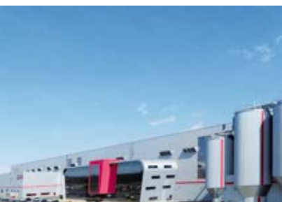
Propapier PM2 plant Eisenhüttenstadt, Germany
