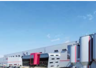
Propapier PM2 plant Eisenhüttenstadt, Germany
