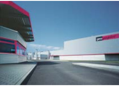
Propapier PM1 plant Burg, Germany
